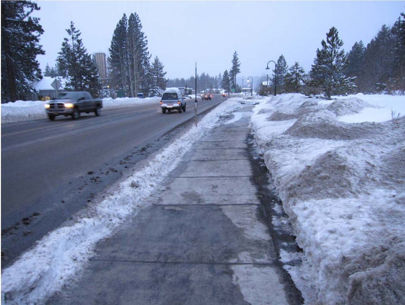
cleared sidewalk along Kingsbury Grade (NV SR207)
