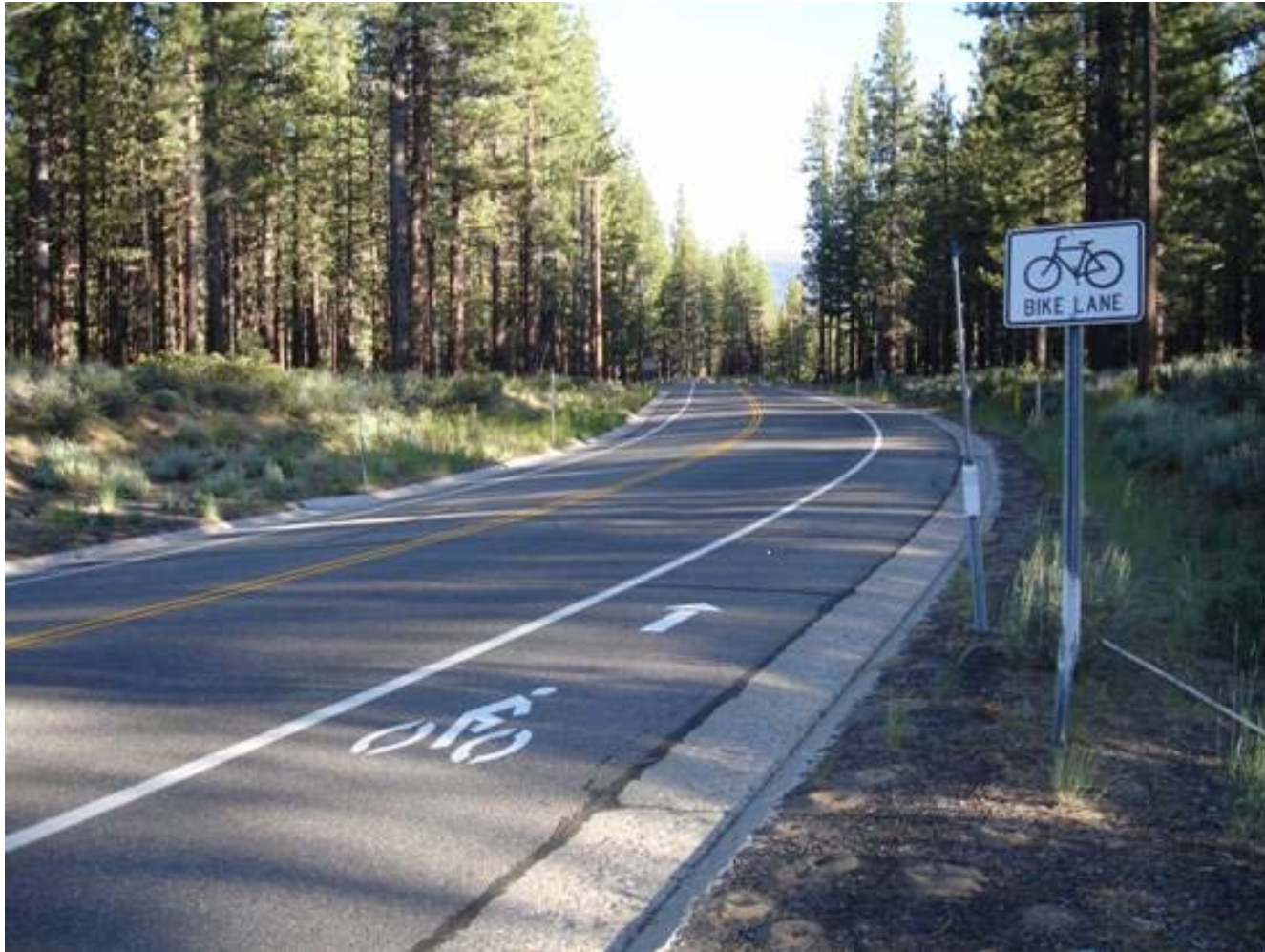
bike lane along Pioneer Trail
