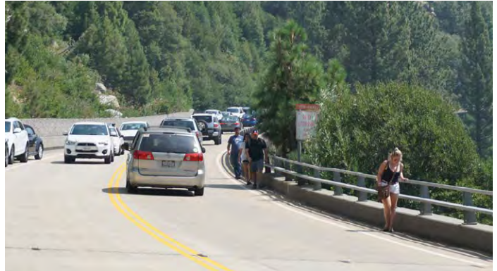
Pedestrians hug the viaduct's guardrail and walk in a 12- to 18-inch shoulder as they walk from their car to their destination.
