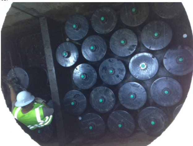
Al Tahoe ECP - Pasadena StormFilter 2013 cartridge replacement AFTER
