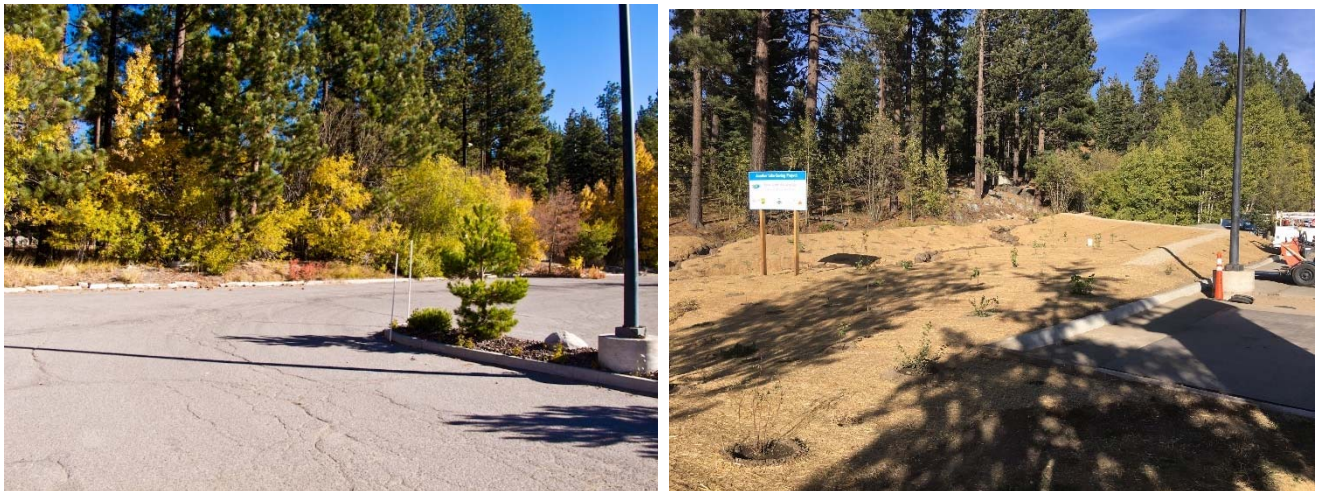
Burke Creek realignment project before (left) and just after realignment (right).
