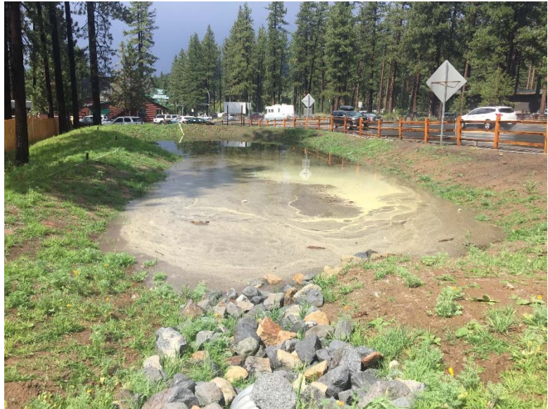
Large infiltration basin to treat stormwater runoff as a part of the Zephyr Cove Water Quality Improvement Project. Photo credit: NTCD
