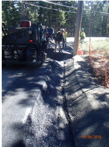
Construction of AC swale on Antelope Way
