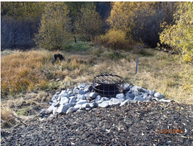
Atrium rack inlet for basin on Fourth Street
