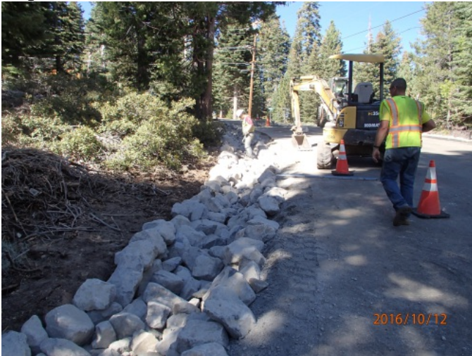
Construction of rock lined channel on Antelope Way
