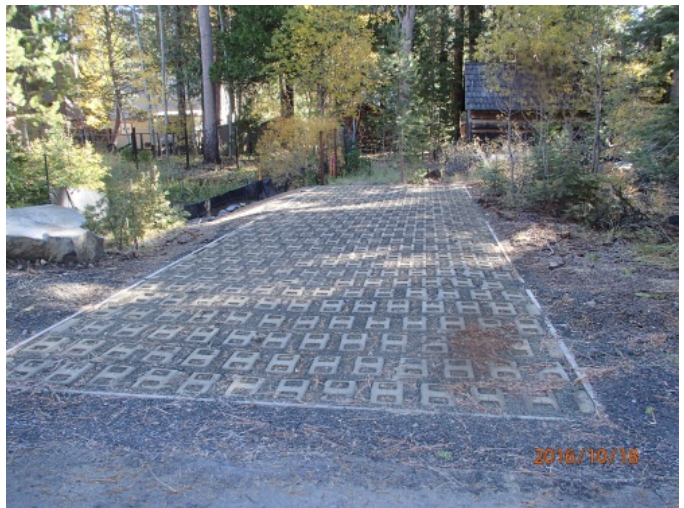
New block pad for vector clean out of Sixth street basin
