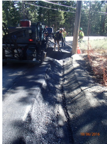
Construction of AC swale on Antelope Way
