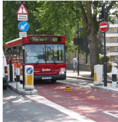
Rising Bollards for Transit
