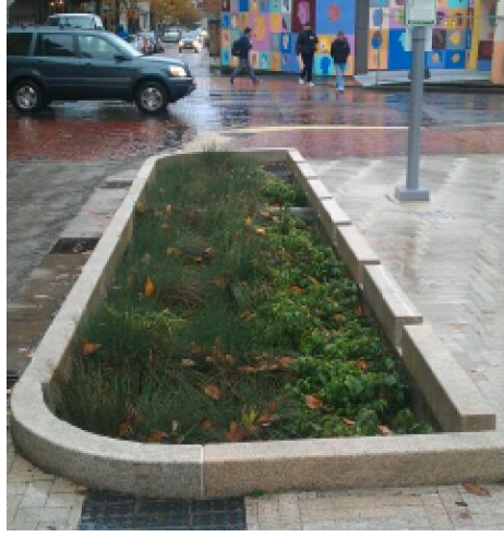
Stormwater Curb Extension
