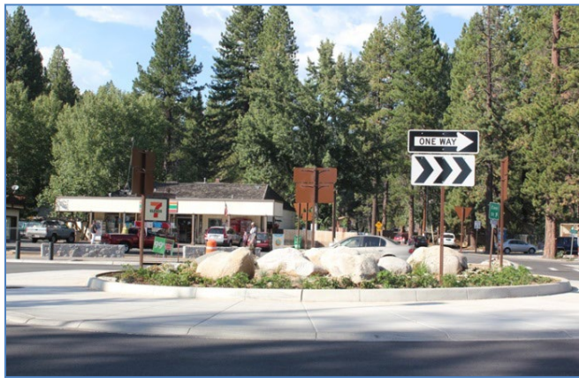
New roundabout in Kings Beach
