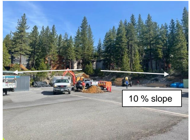
Photo 4 – a. Natural slopes to the north with existing/natural slopes of 8 to 9 percent. 4 b Natural slopes to the east with existing natural slopes of 10 to 11 percent.
