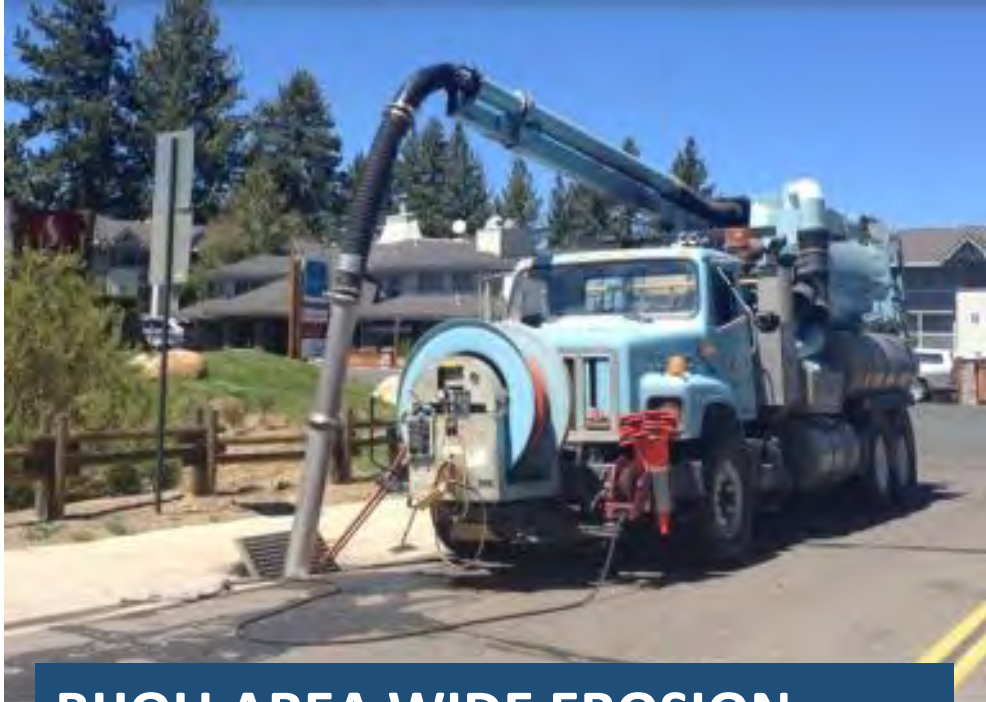
BIJOU AREA WIDE EROSION CONTROL PROJECT
