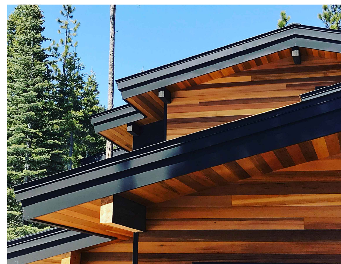
2) METAL ROOFING, METAL FASCIA & SHINGLE MOULD DETAIL. COLOR IS NOT AS PROPOSED. 5) SOFFITS WOOD SIDING IS NOT AS PROPOSED. SEE SCHEDULE.
