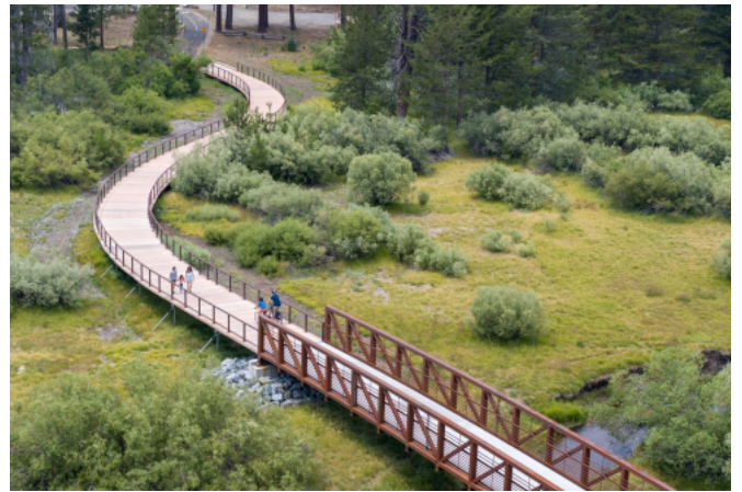
Dennis T. Machida Trail Trout Creek crossing
