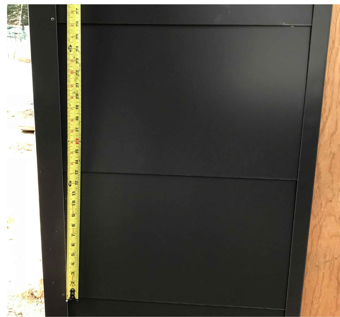
2) METAL PANEL SIDING & TRIM DETAIL. COLOR IS NOT AS PROPOSED - SEE SCHEDULE.
