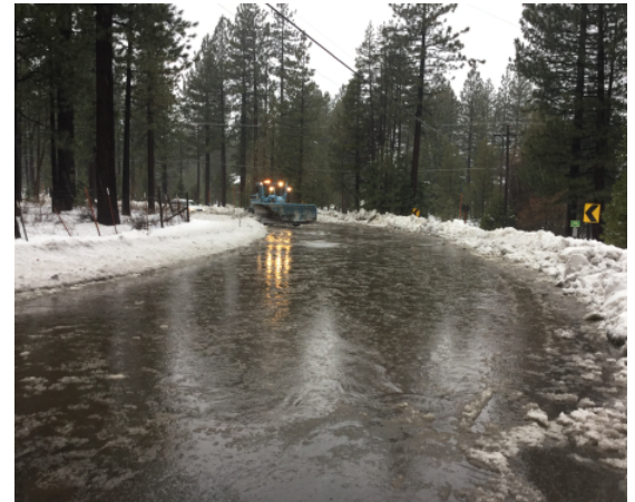
2016- Inadequate drainage creates flooding on South Avenue (major access road to Barton Hospital)
