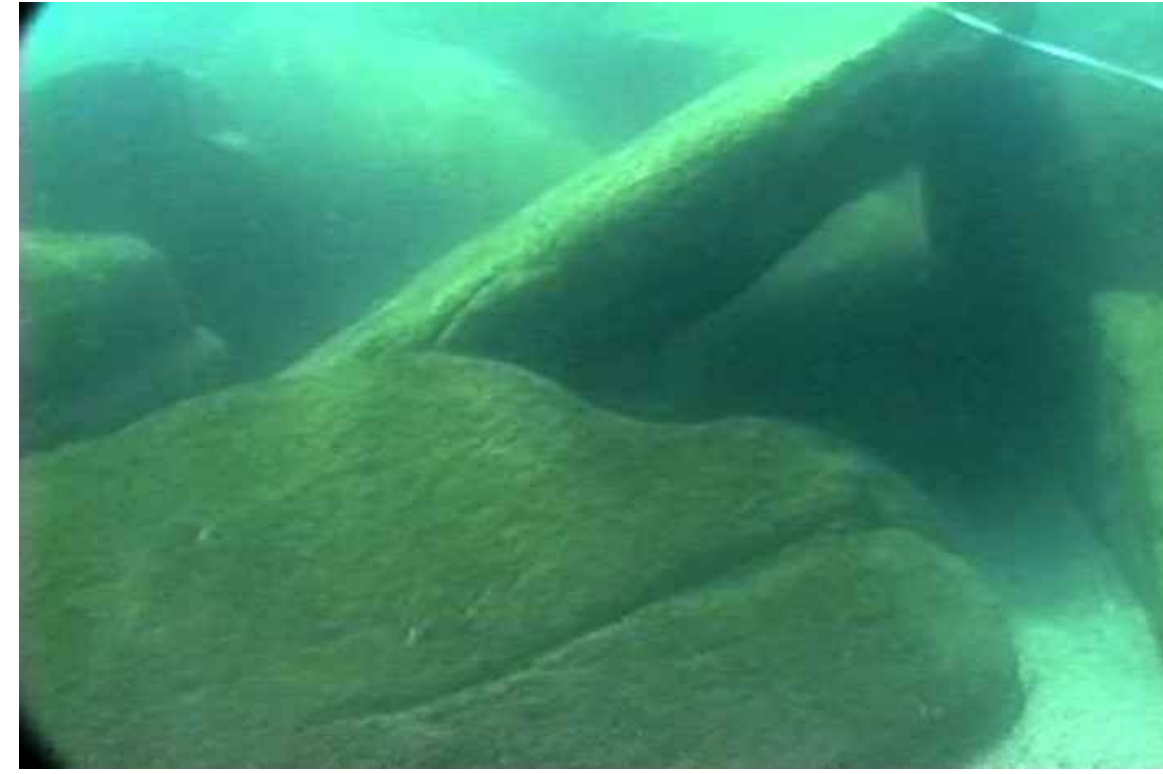
VIEW OF UNDERWATER BOULDERS. NOTE PLATE-LIKE SHAPE AND RANDOM, UNSTABLE ORIENTATION AND BRIDGING.
