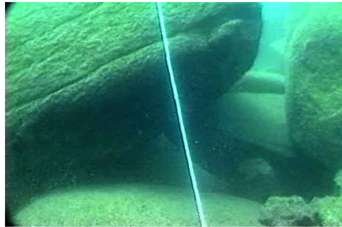
VIEW OF UNDERWATER BOULDERS. NOTE OPENING BENEATH THE BOULDER. TAPE IS APPROXIMATELY 1/2 INCH WIDE.
