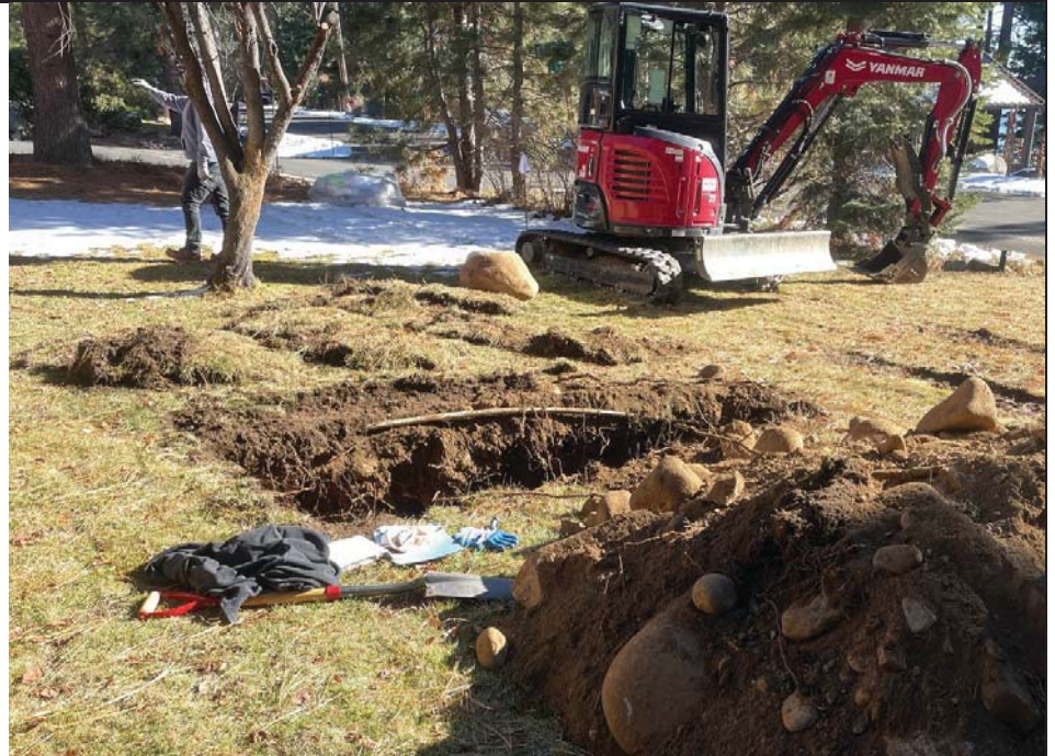
Photo B – View southeast at Test Pit 1, located 25 feet south of residence (deck), 40 feet west of east property line and 35 feet north of south property line. Pit location is representative of parcel and has a 9% slope. The soil layers are composed of mixed colluvium over ancient beach deposit. Profile has 5 to 20% rounded stones and boulders (lower right corner).
