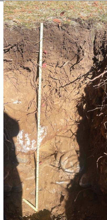
Photo 5 – Close-up view of Test Pit no. 1 showing gravelly-sandy surface layer with many fine and medium roots. Fine roots extend into lower part of profile (60 in. depth). The rockiness of the soil becomes stony and bouldery at 25 inches and increases with depth. These coarse fragments are rounded and smooth, which indicates such area was an ancient shoreline of Lake Tahoe. This soil is unlike the mapped Umpa series, and unlike the Jorge-Tahoma soil types due to the wave-influenced substratum. This is an unnamed inclusion (XXX). For slopes 0 to 16%, this soil rates as Class 6, as per Table 4 of the Bailey land capability system.
