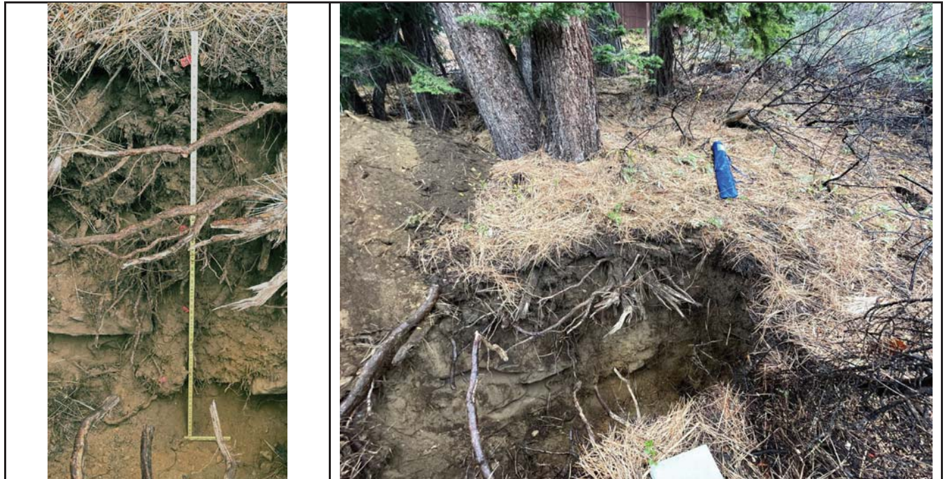
Photo A – View of soil profile showing bottom depth of 46 inches. Fine root penetration to bedrock. No indication of seasonal water table. HSG-B.
