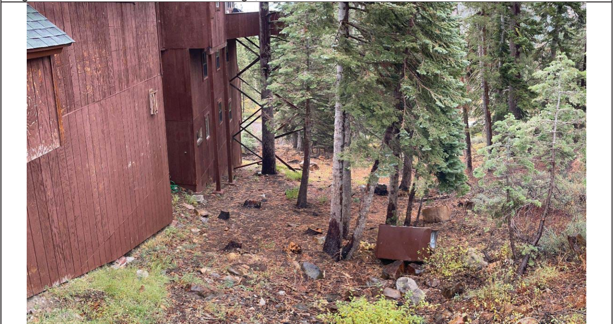
Photo 4 – View to east along west side of residence. This vicinity exhibited more historic ground disturbance, as evident by concrete debris, increased surface stones (side cast during house construction), and less vegetative cover (still no active erosion).
