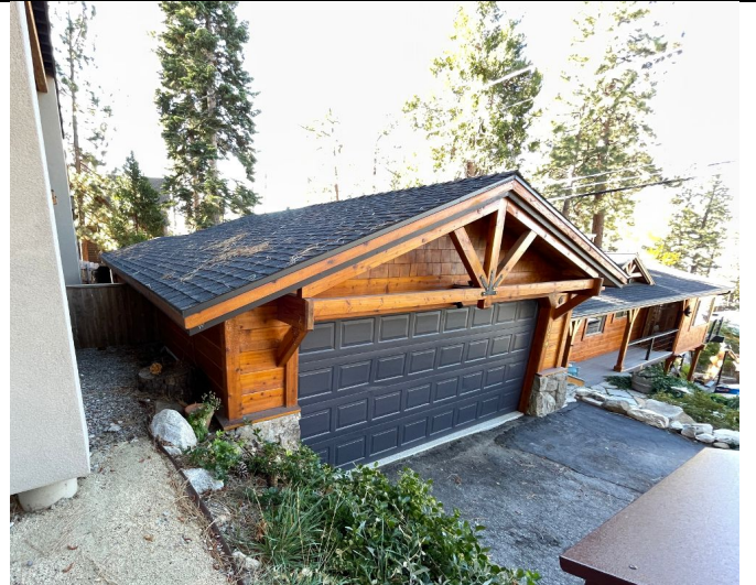
Photo 9. View southwest at east edge of garage which abuts the property line.
